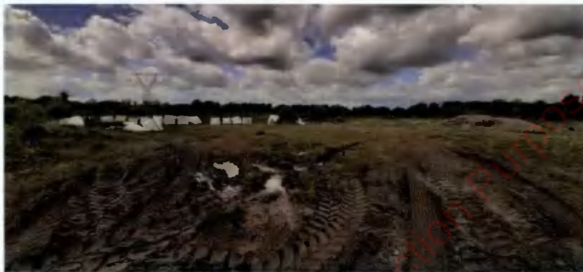
Figure 5-11. Image showing the skip sacks at the eastern side of the central pond. Pile of wood chippings is visible on the right hand side of the image.
